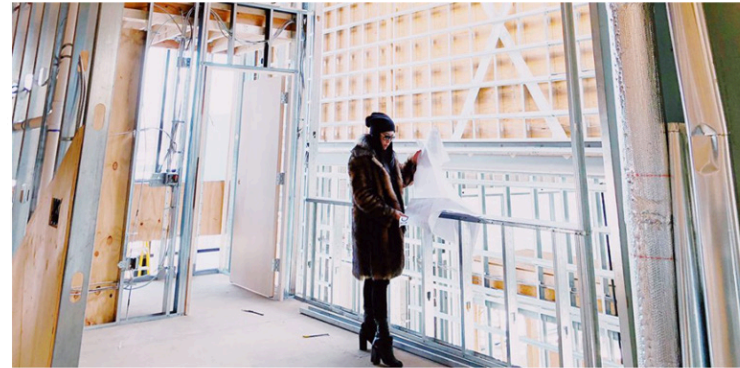
Design Army co-founder and Chief Creative Officer Pum Lefebure checks on the construction progress of At Yolk in Washington, D.C.
